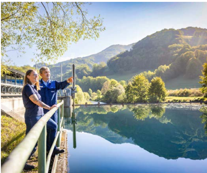
GF operates a hydroelectric power plant on its premises in Traisen (Austria) to generate electricity for its own use.
